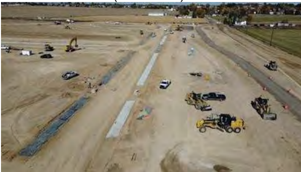
Muturu Road (View: North)
