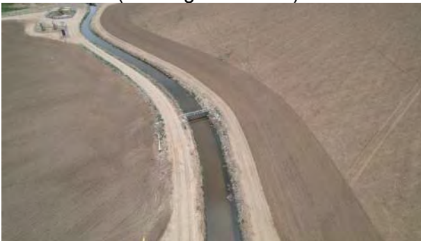
Ditch Realignment Near North End of Site (Looking Northeast)
