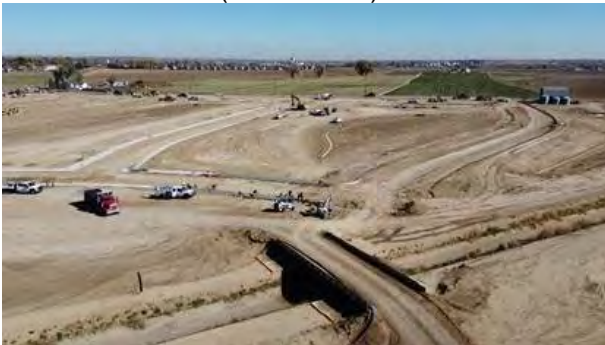
Temp Bridge Over Ditch Near Roosevelt Pkwy. (View: East)
