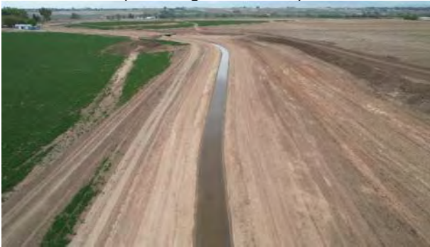
Ditch Realignment (Looking Northwest)
