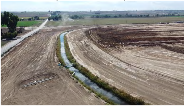
Ditch Realignment southeast of bridge (View: South)
