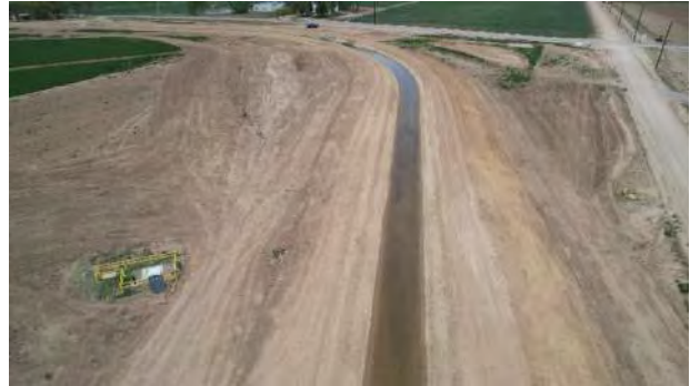
Ditch Realignment Adjacent to CR 46 (Looking East)
