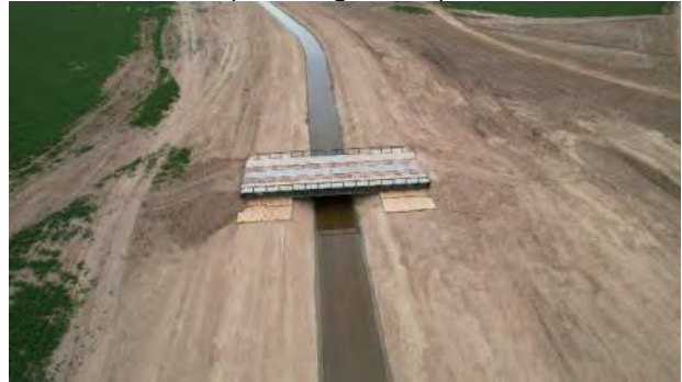
Temporary Bridge over Ditch Realignment
