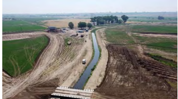
Ditch Realignment northeast of bridge (View: South)
