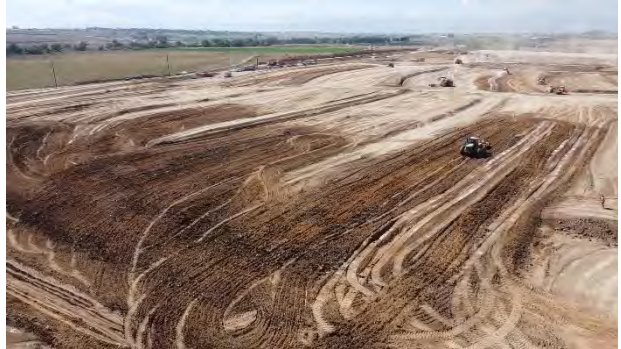
Mass Grading on site (View: Southwest)
