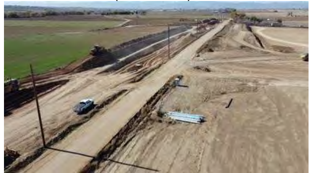
County Road 46 Waterline Improvements (View: Southwest)
