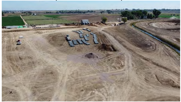
Northern end of Ditch Realignment (View: Southeast)
