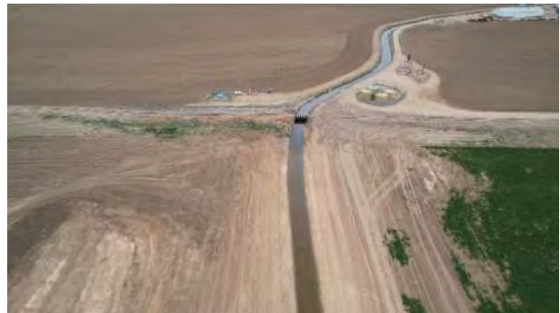
Ditch Realignment at North End of Site (Looking North)
