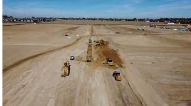
Galloway Drive Utility Improvements (View: North)
