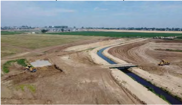
Ditch Realignment southwest of bridge (Looking Northwest)
